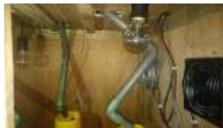
Figure 11. Placement Of Hardware in The Cage
