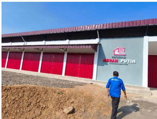
Figure 2. Merah Putih Cooperative facility in Karangpaningal Village, Tambaksari District, Ciamis Regency
